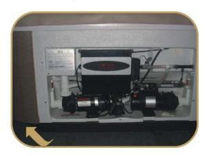
6. Check the pump unions (circled in illustration) to be sure they are hand tight to prevent the possibility of leakage.
