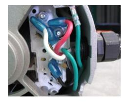
**4. For 1 speed pumps** you will not have a red wire on your pump amp cord. Follow the motor wiring diagram for the black 1 speed.
