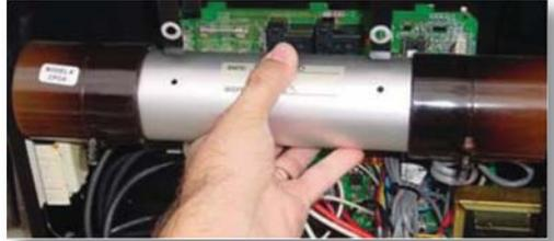
9. Place new UltraPure Ozone Generator Assembly in location of old unit. Line up screw indents on the tube with mounting strip holes, for easy installation. You will need to hold the tube assembly carefully from behind to insure it does not push against any other electrical components and cause breakage. Carefully install mounting screws into new tube assembly using a cordless drill. The aluminum tube is thick and using a hand screwdriver will be very slow.
