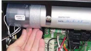
10. To attach vinyl hose to the correct barbs, putting a little soapy water on the plastic barbs before sliding the hose on can help. The soapy solution acts as a lubricant.
