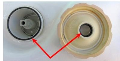
**Step 5:** Using a Scotch Brite Pad, or other abrasive sponge, wipe the inside of the valve housing and diverter. Once the area is clean, reassemble the valve - reinsert the diverter, screw on the threaded cap, then replace the knob.
