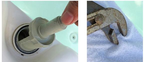
**Step 4:** There are two O-rings that seal the threaded cap to prevent water from leaking out the top of the assembly. Check these rings to see if they are worn or degrading. If they are, call us to order a new set. (01510-73 large / 01522-56 small)
