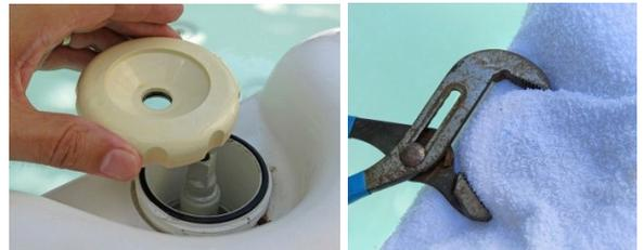
**Step 3:** Grasp the diverter stem and pull it straight out of the valve housing. If it is difficult to remove, use your channel-lock pliers and a towel again to pull it out. If it still won't come out, please call us; we have a trick that will help.
